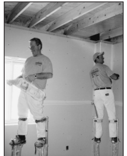
Drywall taping.
